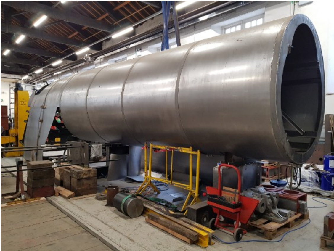
Progress on the cladding - Mandy Grant
